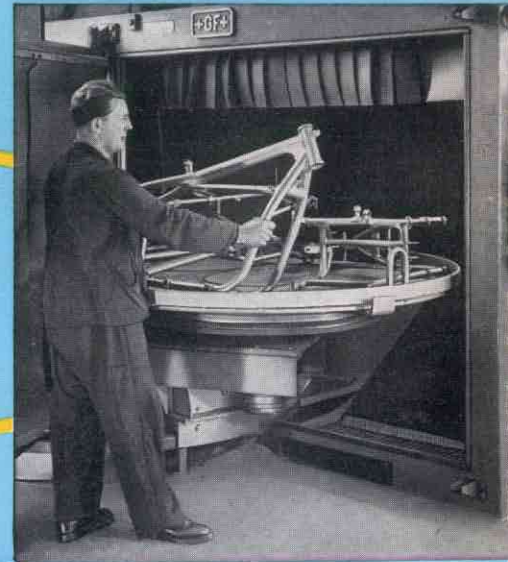
Modern sand blasting equipment, ensures a good paint finish.
